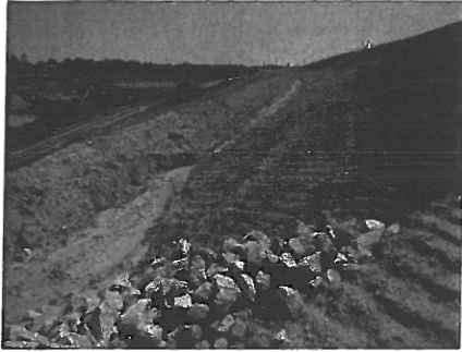
5/22/15, photo 20 of diversion berm on Section IV
